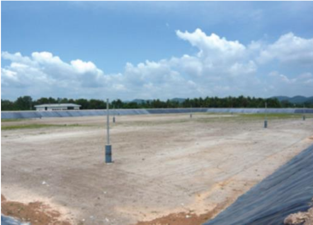
Figure 4 The trench method
